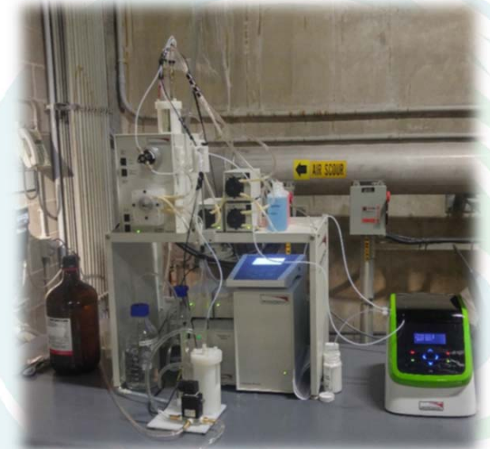
Online pH, Conductivity, and COD Installed on Rolling Cart for use at different plant locations
